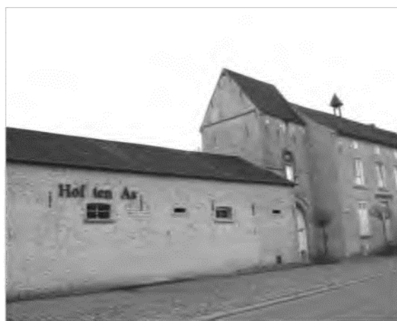
De vroegere paardenstalling genaamd "De Quade Plas", nu Hof Ten As
